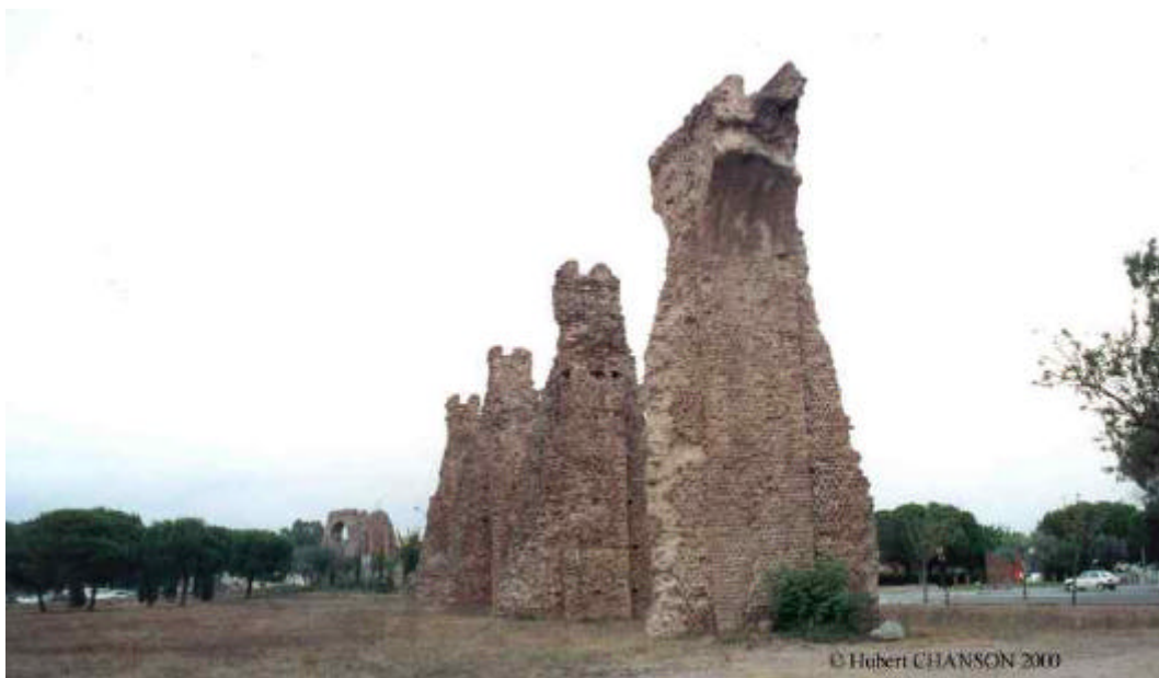
(E) Fréjus aqueduct (France)- Arches de Sainte Croix, looking upstream on 14 Sept. 2000 - The open channel conduit was at the top of the arcades
