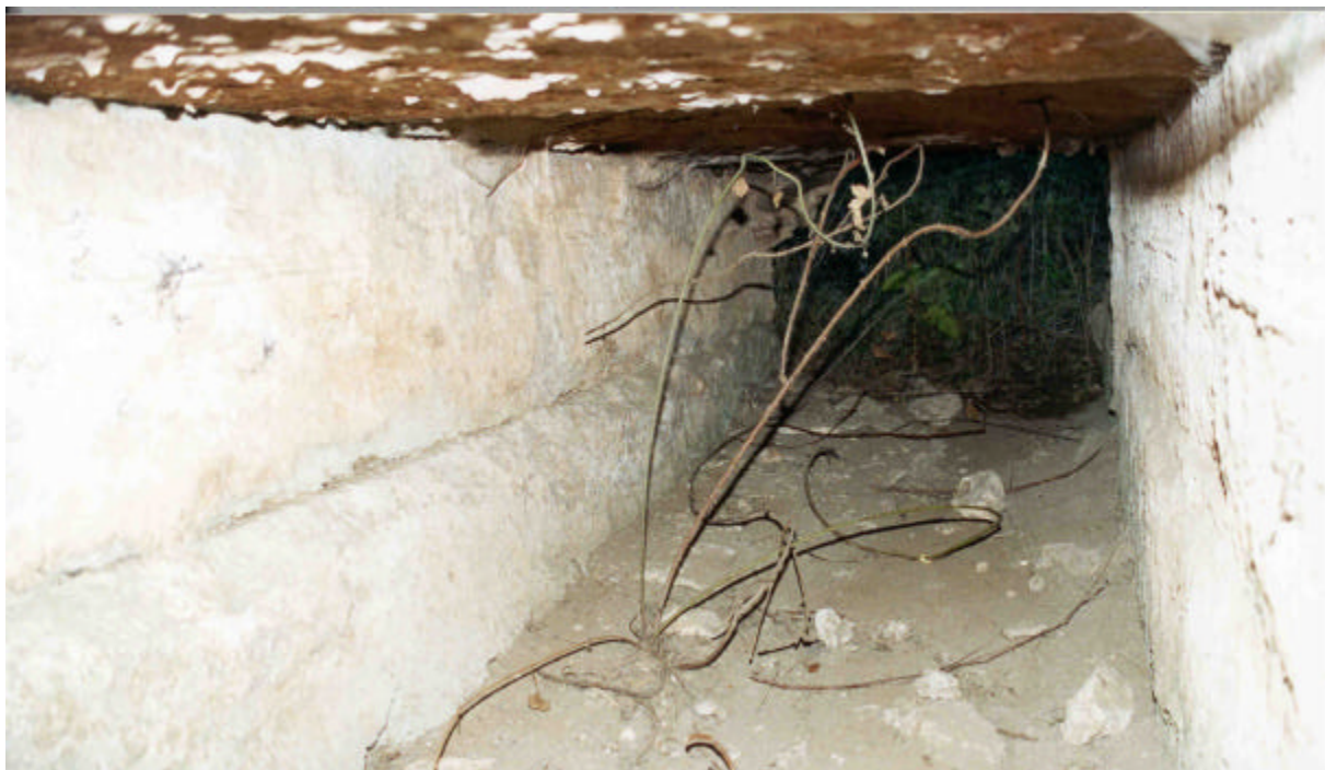
(C) Culvert beneath the aqueduct between Combe de Sartanette and Combe Saint Joseph, downstream of Pont du Gard in Sept. 2000 - Main culvert cell (0.8-m wide)
