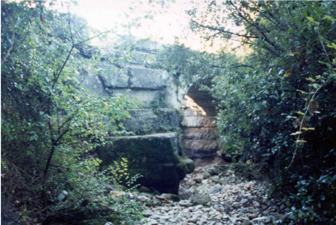
(C) Culvert beneath the aqueduct between Combe de Sartanette and Combe Saint Joseph, downstream of Pont du Gard in Sept. 2000 - Main culvert cell (0.8-m wide)
