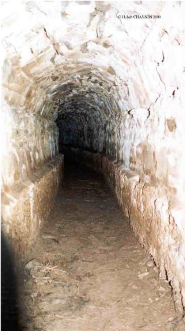
(C) Brévenne aqueduct, Lyon, France (70 km long) - Biternay in Sept. 2000, inside the conduit, looking upstream
