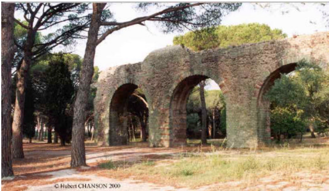
(E) Fréjus aqueduct (France)- Arches de Sainte Croix, looking upstream on 14 Sept. 2000 - The open channel conduit was at the top of the arcades
