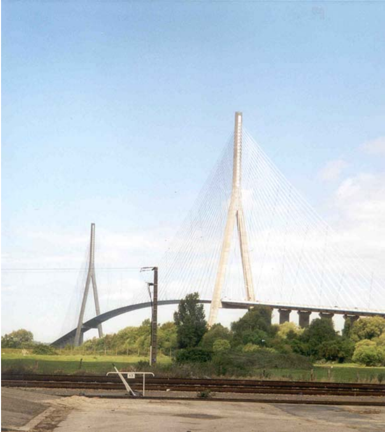
Fig. 1-3 - Le Pont de Normandie (France) in May 2003 (A) View from the South in May 2003 (Courtesy of Mr and Mrs CHANSON)
