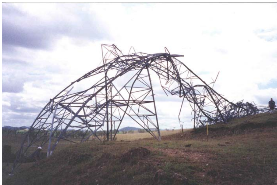
(B) Damaged transmission tower (275 kV double circuit electricity transmission tower)
