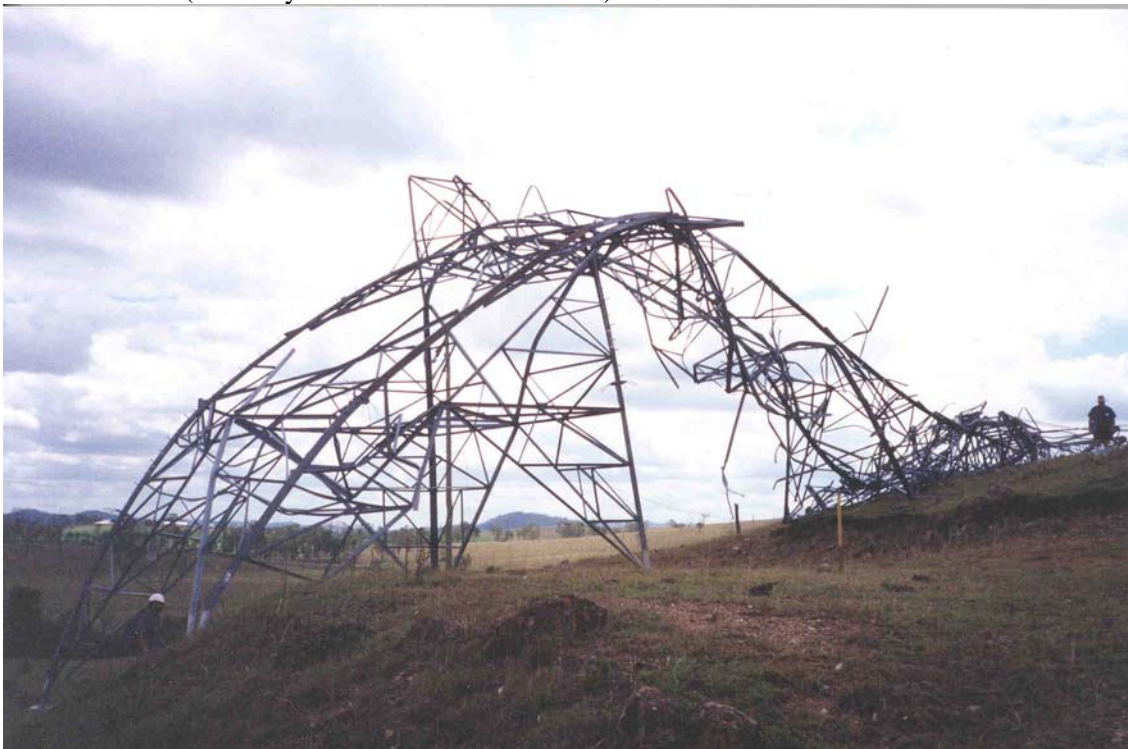
Fig. 1-1 - Damaged transmission tower (275 kV double circuit electricity transmission tower) in the Brisbane valley in March 1998 (Courtesy of Prof C. LETCHFORD)
