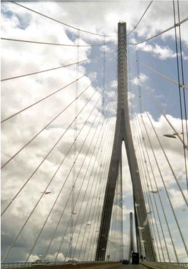
Fig. 1-3 - Le Pont de Normandie (France) in May 2003- North pier, driving South (Courtesy of Mr and Mrs CHANSON)
