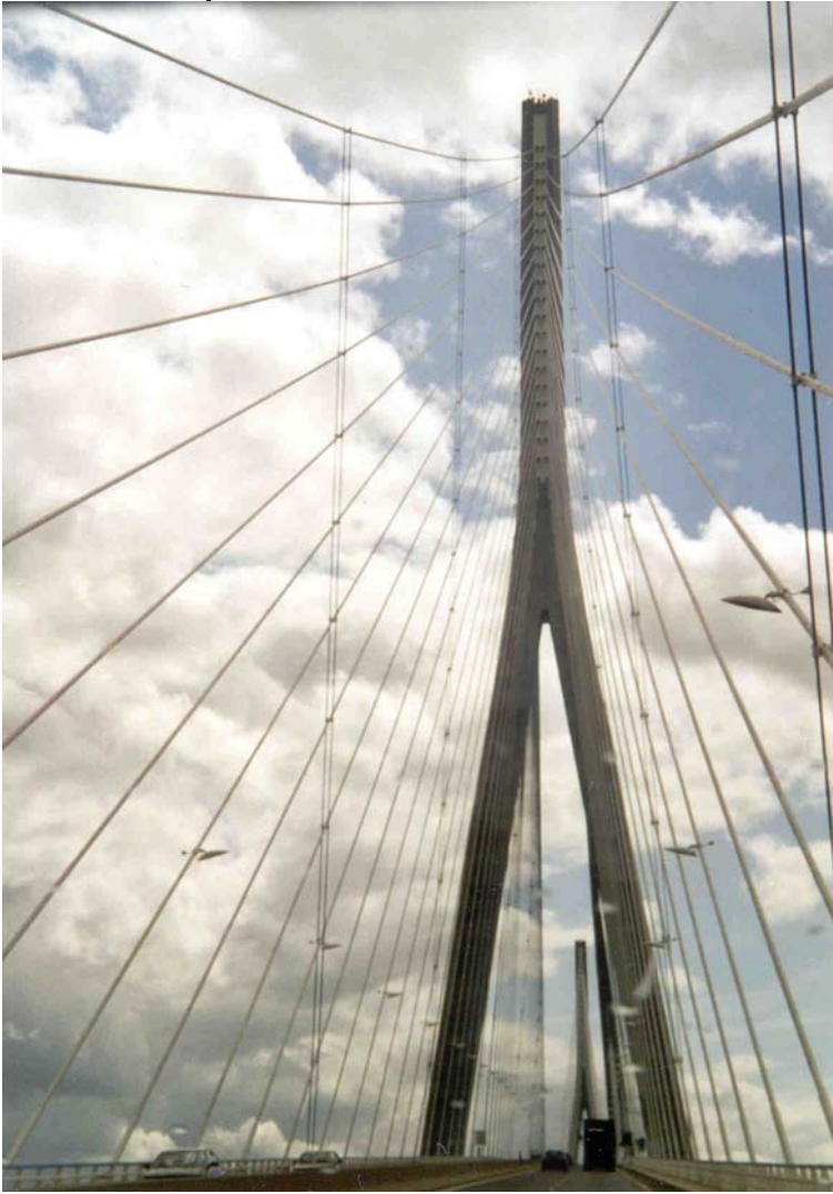
(B) North pier, driving South (Courtesy of Mr and Mrs CHANSON)
