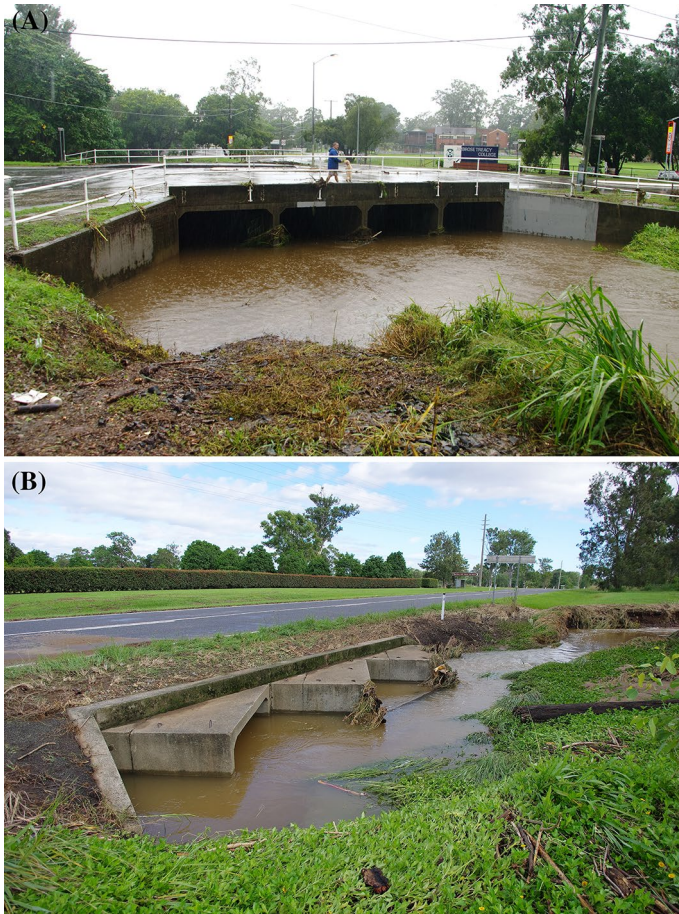
Fig. 1 Box culvert operation. A Box culvert outlet on 30 March 2017—stream; Whitton Creek, Brisbane QLD (Australia)—flow direction from background to foreground. B Box culvert inlet operation on 31 March 2017 for less-than-design flow conditions—stream: Caswell Creek, Canungra QLD (Australia)—flow direction from background right to foreground left
