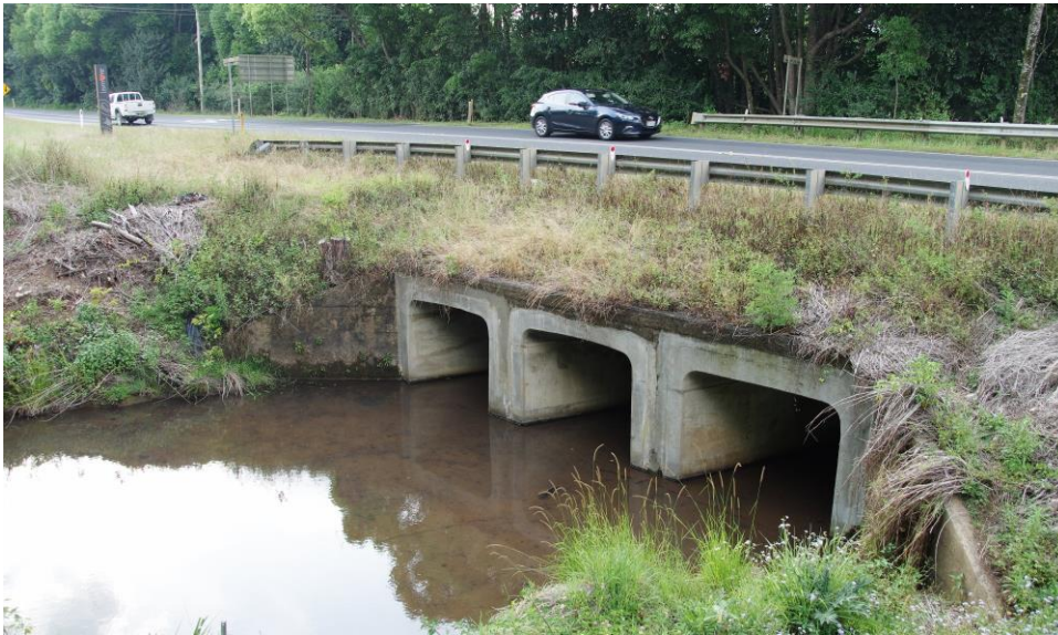
Figure 1 – Three-cell standard box culvert outlet along Marom Creek beneath Bruxner highway B60, at Wollongbar NSW (Australia) on 28 October 2016.
