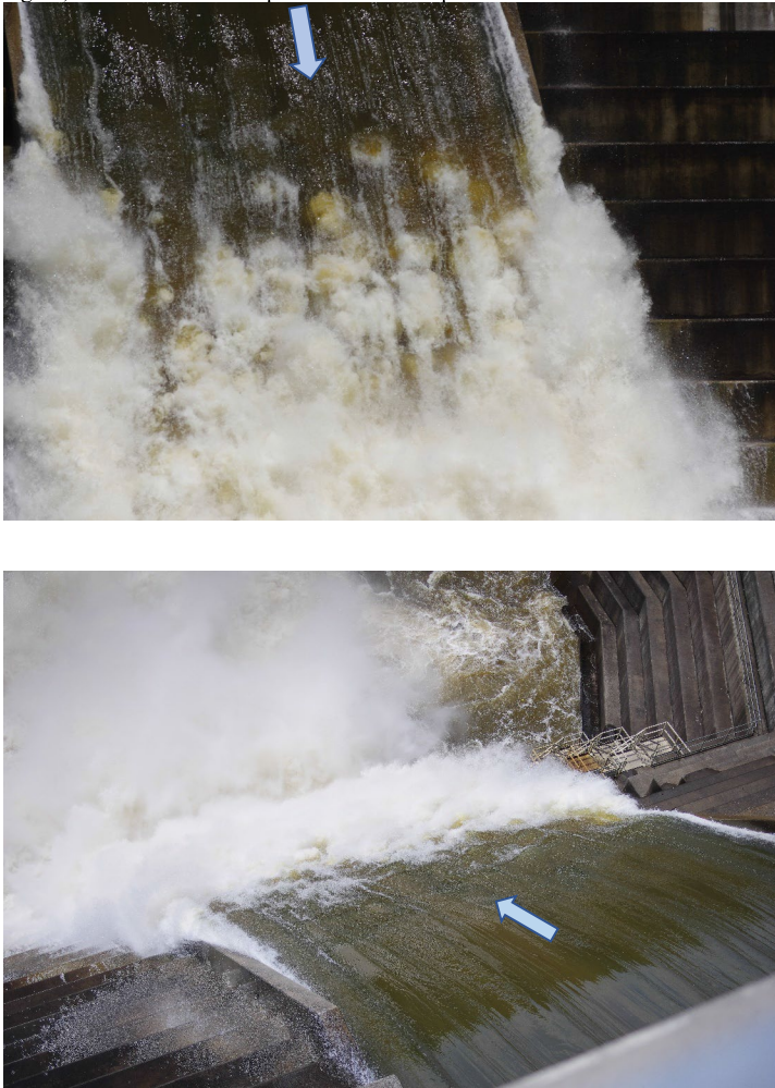
Fig. 1 Onset of self-aeration on overflow spillways
