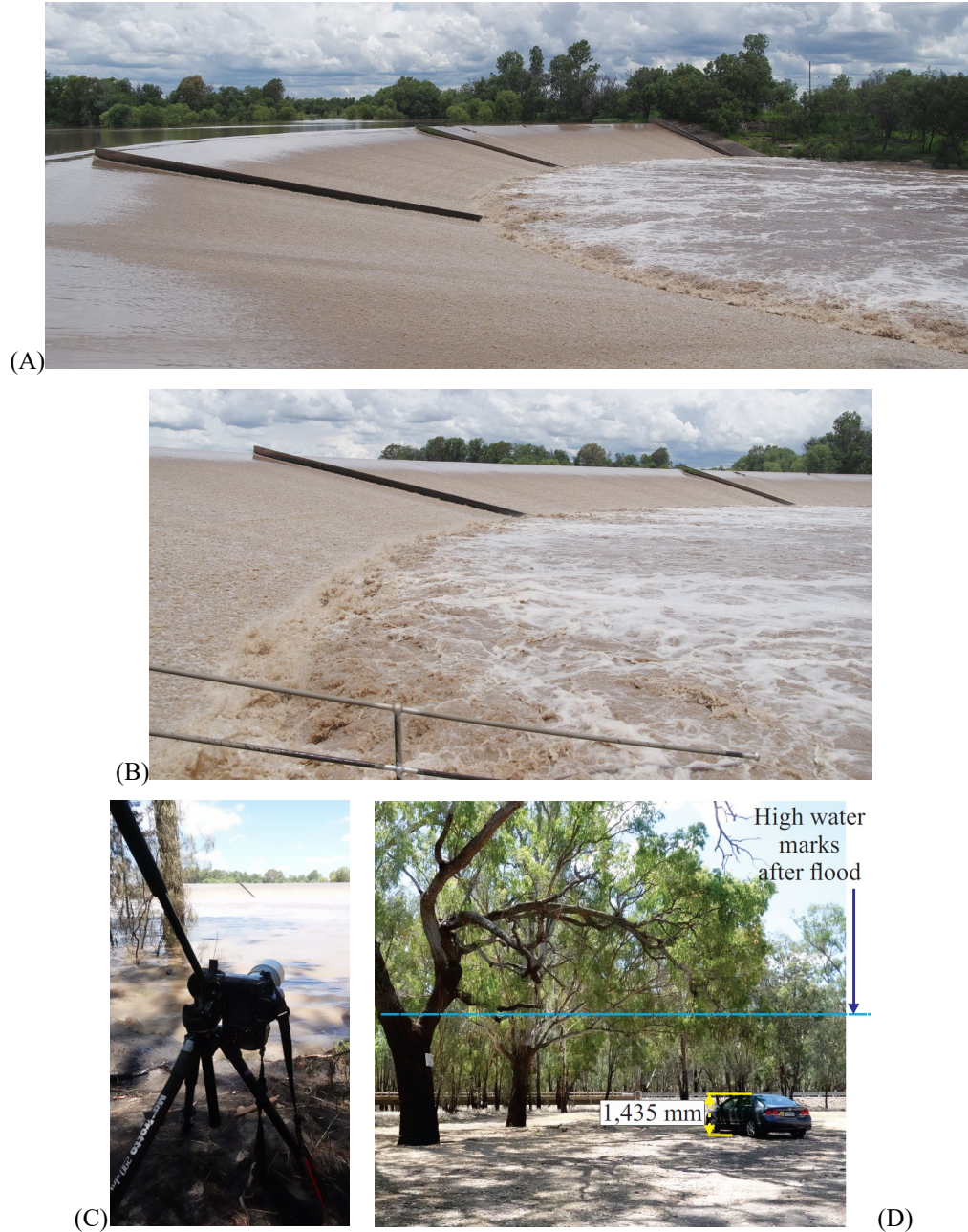
Figure 2. Chinchilla Minimum Energy Loss (MEL) weir (QLD, Australia). (A) Overflow on 27 November 2021 ( Q = 121 \text{ m}^3/\text{s} ); (B) Hydraulic jump at the chute toe on 27 November 2021 ( Q = 121 \text{ m}^3/\text{s} , Shutter speed: 1/2,500 \text{ s} ); (C) Camera tripod setup on the lower right bank; (D) High-water marks on the right bank on 15 December 2021
