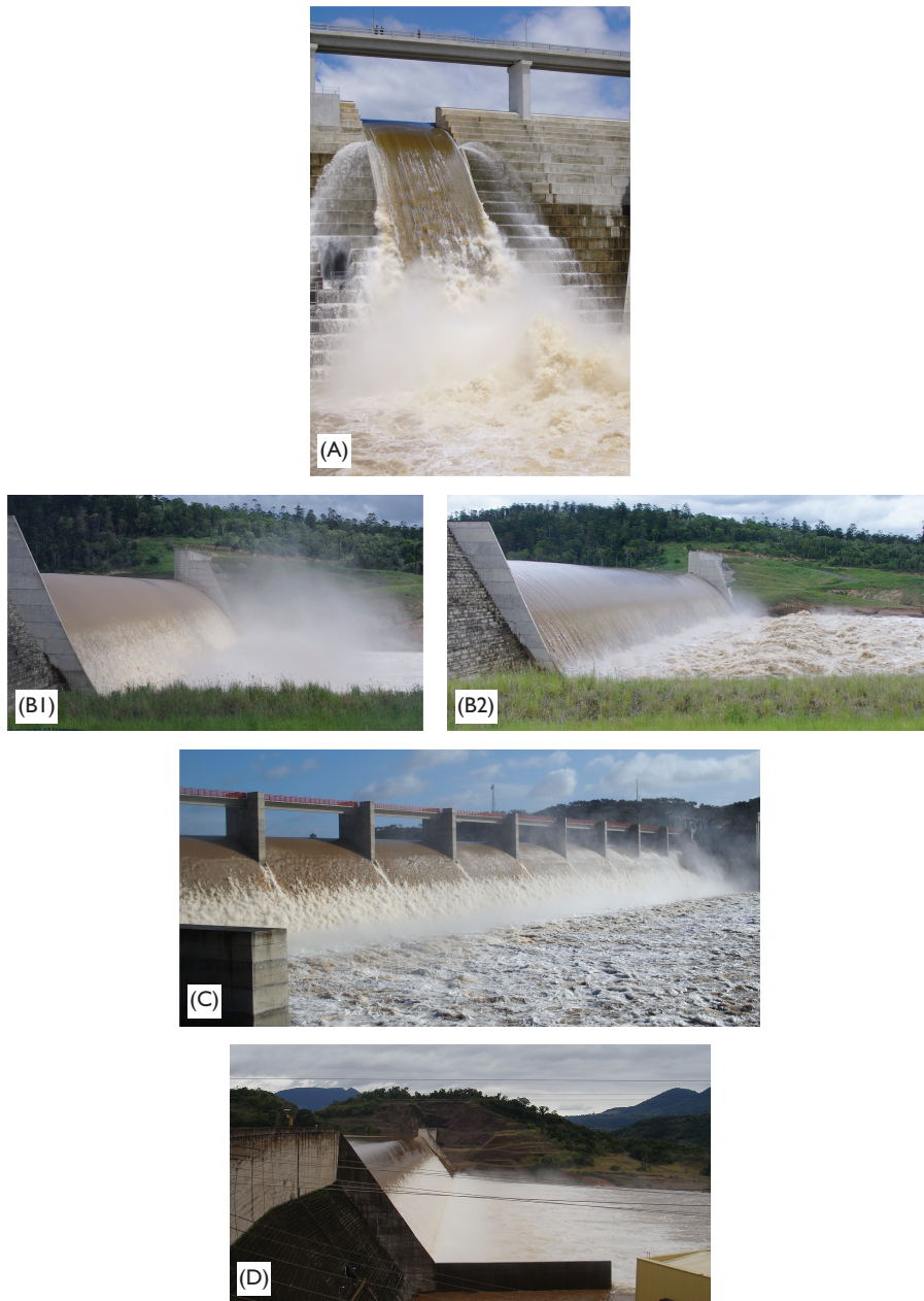
Figure 3.10 Prototype stepped spillway operations. (A) Hinze dam spillway ( \theta = 51.3^\circ , h = 1.2 m, Q = 200 m 3 /s, d_c/h = 2.5 on 29 Jan. 2013). (B1) Paradise dam spillway ( \theta = 57.4^\circ , h = 0.62 m, Q = 2,320 m 3 /s, d_c/h = 2.85 on 5 Mar. 2013). (B2) Paradise dam spillway ( \theta = 57.4^\circ , h = 0.62 m, Q = 6,000 m 3 /s, d_c/h = 5.4 on 30 Dec. 2010). (C) Pedrógão dam ( \theta = 53.1^\circ , h = 0.6 m, on 10 Jan. 2010) (Courtesy of EDIA). (D) Dona Francisca dam ( \theta = 53.1^\circ , h = 0.6 m, in July 2011) (Courtesy of Marcelo Marques).
