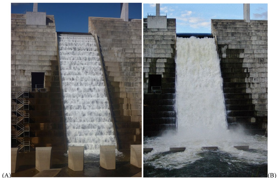
Fig. 2 Hinze Dam stepped spillway, Australia during low overflows, h=1.5 m, 1 V:0.80H slope— A q=0.062 m 2 /s, d_c/h=0.04 , Re=2.5\times 10^5 , nappe flow regime on 25 April 2013 (Photograph Davide Wüthrich); B q=1.7 m 2 /s, d_c/h=0.45 , Re=6.8\times 10^6 , transition flow regime on 3 May 2015 (Photograph Hubert Chanson)
