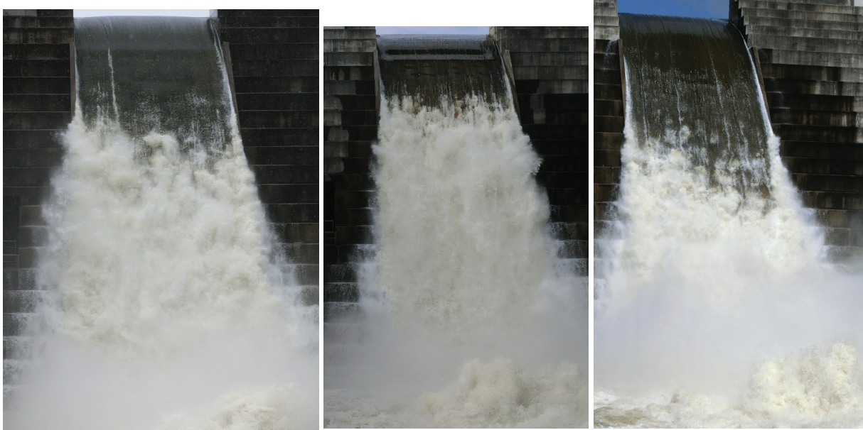
Figure 2. Hinze dam stepped spillway (Australia) in 2021, h = 1.5 m, 1V:0.8H slope - From left to right: d_c/h = 1.0 (27 March 2021), shutter speed: 1/2,000s; d_c/h = 1.35 (23 March 2021), shutter speed: 1/1,000s; d_c/h = 1.58 (24 March 2021), shutter speed: 1/2,000s.
