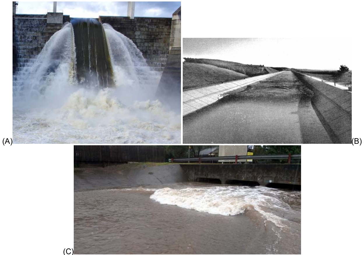
Figure 1. Challenges in hydraulic structure design. (A) Self-aeration at the Hinze dam spillway on 31 March 2017 ( d_c/h = 3.55 , Re = 1.1 \times 10^8 ); (B) Transient positive surge propagating in the Oraison hydropower canal following a rapid stoppage ( Q = 210 \text{ m}^3/\text{s} , Re \sim 10^7 ) (Photo I.G.N. in Cunge 1966); (C) Standard box culvert operation on Cubberla Creek on 4 June 2016, with a hydraulic jump in the inlet (Courtesy of Stewart Matthews)
