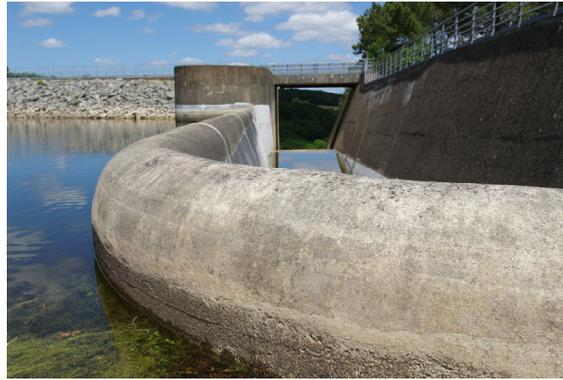
**Figure 1. Circular-crested weir application: half-round crest along the lateral spillway of Chèze dam (France) on 11 June 2022.**
