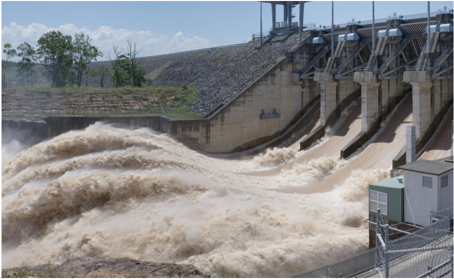
Fig. 3 Wivenhoe Dam spillway ski jump (Australia) during operation on 17 January 2011 at 13:20 (local time)—note the large amount of entrained air in the spillway flow and at the jump take-off
