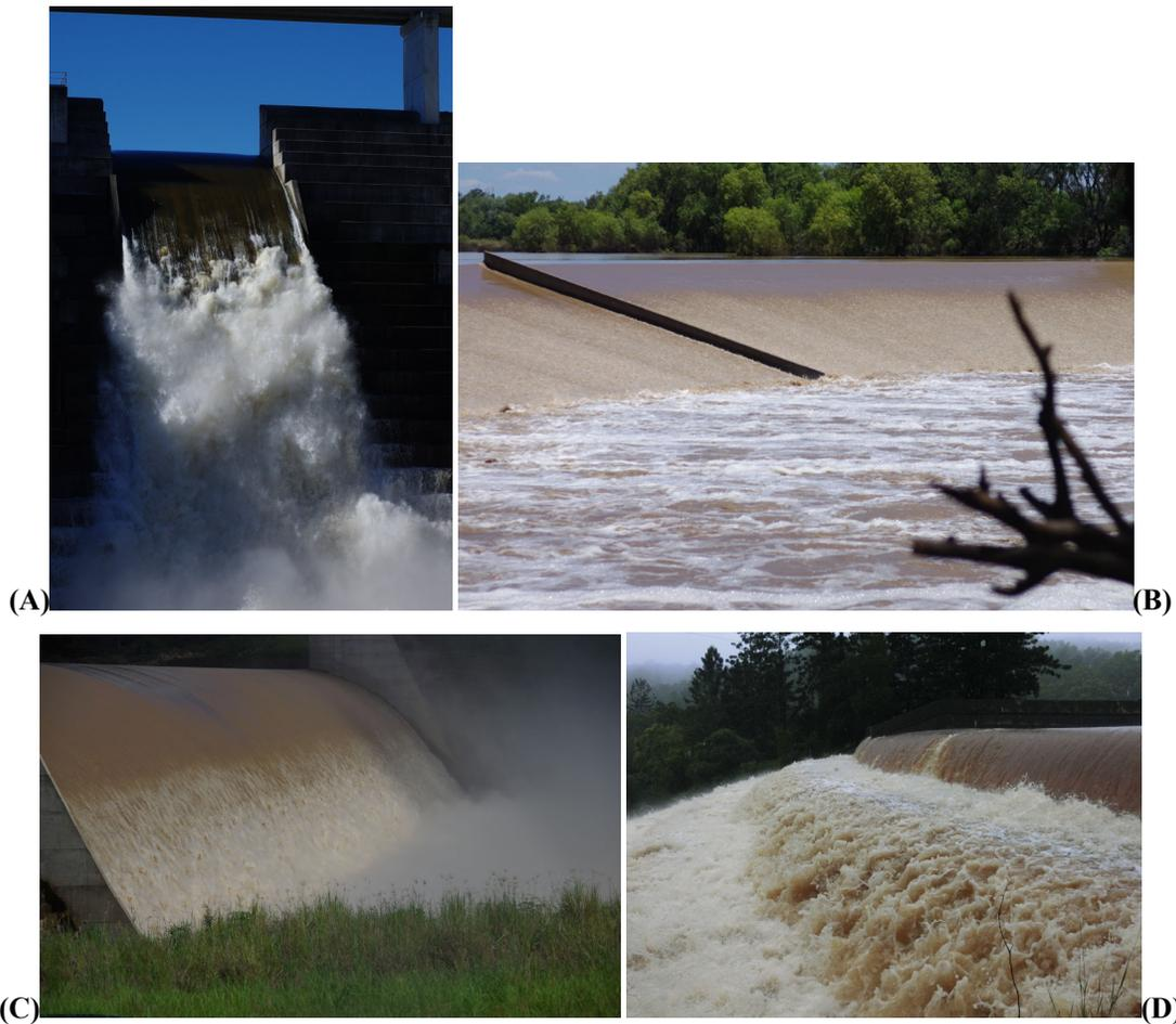
**Figure 1. Large dam spillway operations in Queensland (Australia). (A) Hinze Dam Stage 3 on 5 March 2022 ( $Q = 85.5 \text{ m}^3/\text{s}$ ). (B) Chinchilla MEL weir on 15 Dec. 2021 ( $Q = 144 \text{ m}^3/\text{s}$ ). (C) Paradise Dam on 5 March 2013 ( $Q = 2,500 \text{ m}^3/\text{s}$ ). (D) Gold Greek Dam on 26 Feb. 2022 ( $Q = 38 \text{ m}^3/\text{s}$ ).**
