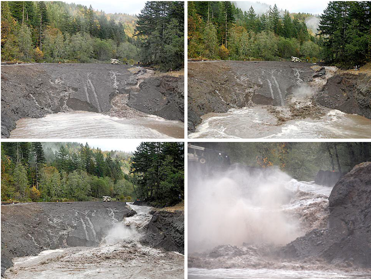
Fig. 4 Embankment breaching. a Marmot Dam cofferdam breaching (USA) on 19 October 2007 (Courtesy of Portland General Electric)—the cofferdam was built as part of the Marmot (concrete) dam removal to restore fish migration along the Sandy River, b physical modelling of non-cohesive embankment dam failure at the University of Auckland in 2012— H = 0.3 m, L = 1.5 m, d_{50} = 0.3 mm, constant upstream head experiment—flow direction from left to right with the reservoir on the right —the first five shots (1–5) were taken during the breach development; the last two shots (7–8) show details of the breach after the reservoir draining
