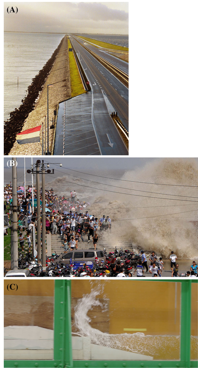
Fig. 2 Examples of river and coastal embankments. a Coastal barrier in Netherlands: Zeidersee enclosure dam (Courtesy of Ronald De Heer), b tidal bore of the Qiantang River (China) overtopping a river dyke on 31 August 2011, c physical model of a coastal barrier during a tsunami—physical test with tsunami wave model propagating from right to left and impacting the embankment
