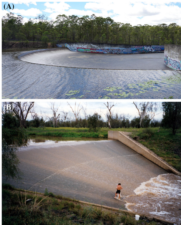
Fig. 6 Minimum energy loss (MEL) spillway and weir. a Minimum energy loss spillway inlet of Lake Kurwongbah (Brisbane, Australia) in operation on 29 January 2013, b lemontree minimum energy weir (Australia) on 8 November 1997 for a small discharge ( Q \ll Q_{des} )
