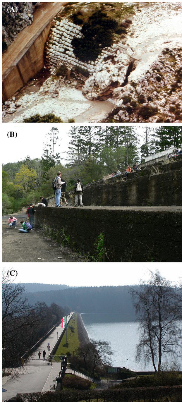
Fig. 1 Examples of embankment dam structures. a Embankment dam with overtopping stepped spillway: stepped weir in Akarnania (Greece) (Courtesy of Professor Knauss)—completion: BC 1,300, H = 10.5 m, L = 25 m, b concrete stepped spillway of Gold Creek dam (Australia) with the embankment dam in the background—completion: 1885, H = 26 m, L = 187 m—the concrete spillway was built over the right abutment, c embankment dam: Sorpe dam (Germany) on 31 March 2004 viewed from left bank—completion: 1935, H = 69 m, L = 700 m
