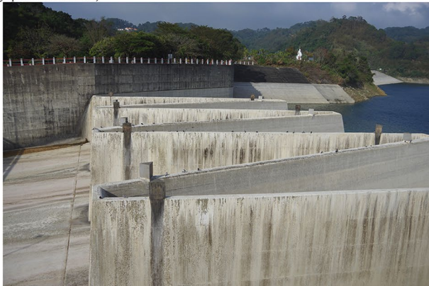
(G) Labyrinth weir at the crest of the Shilin Dam spillway, on the Daan River (Taiwan) on 9 January 2016 (Photograph H. CHANSON)
