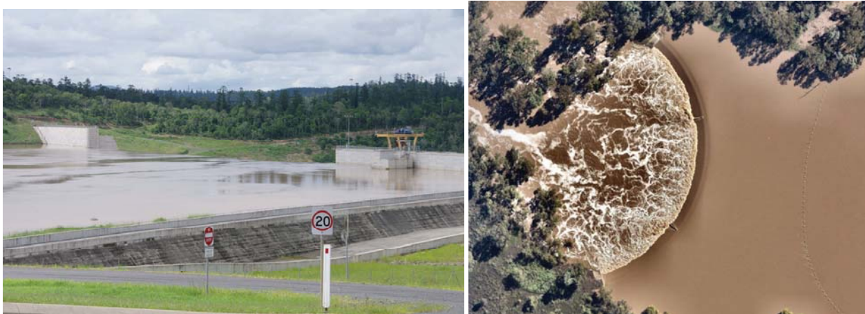
Figure 3. Approach flow conditions at Paradise Dam and Chinchilla weir during major flood operations. Left: Paradise Dam on 30 December 2010 for Re = 7.5 \times 10^5 ; Right: Chinchilla weir on 6 April 2022 for Re \sim 6 \times 10^6 (Photo NearMap).
