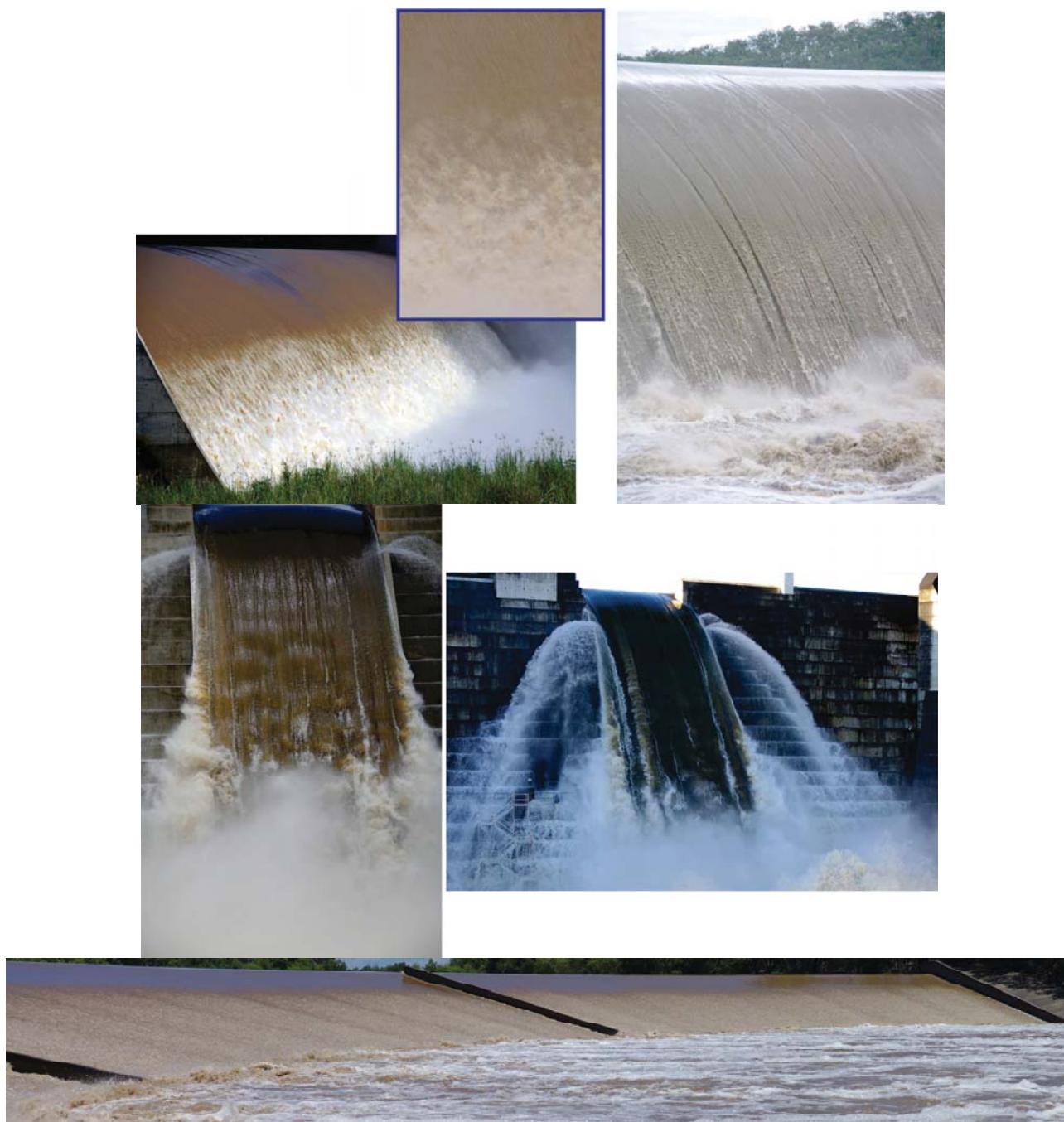
Figure 2. Self-aeration at prototype spillways during major flood operation. Top: Paradise Dam spillway for Re = 2.9 \times 10^7 (Left) and 7.5 \times 10^7 (Right). Middle: Hinze Dam spillway for Re = 6.5 \times 10^7 (Left) and 8.1 \times 10^7 (Right). Bottom: Chinchilla weir for Re = 2.7 \times 10^6 / 4.6 \times 10^6 . All photographs are high shutter speed with exposure time < 1 ms.
