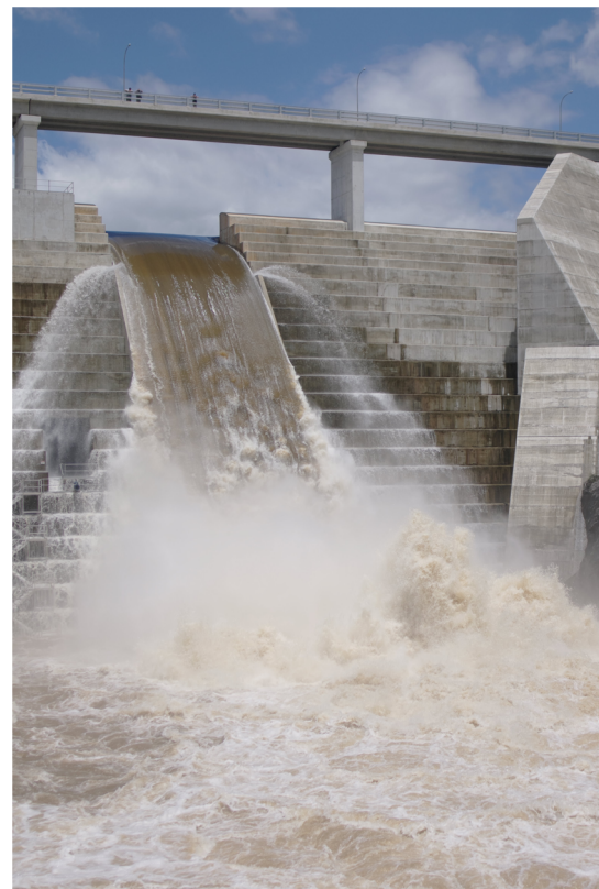
Fig. 2. Hinze Dam stepped spillway (Australia) in operation (spillway geometry: \alpha = 51.3^\circ , h = 1.2 m, rockfill dam wall with conventional concrete spillway): view from downstream for q = 14 m 2 /s on January 29, 2013 (shutter speed: 1/8,000 s)
