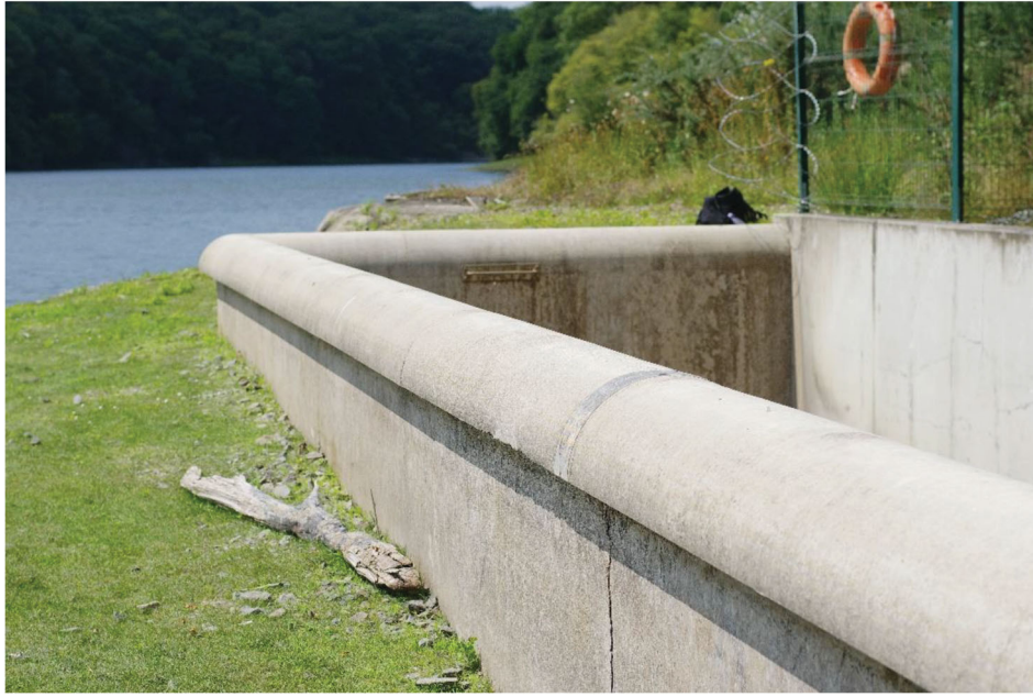
Figure 1. Half-round circular crested weir at Barrage de Pont Ruffier (France) on 2 August 2024.
