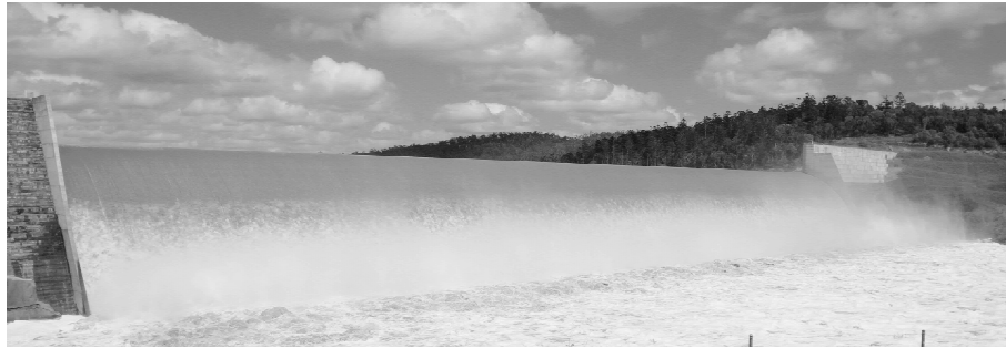
Figure 2. Strong turbulence and intense free-surface aeration in a skimming flow on a stepped spillway
