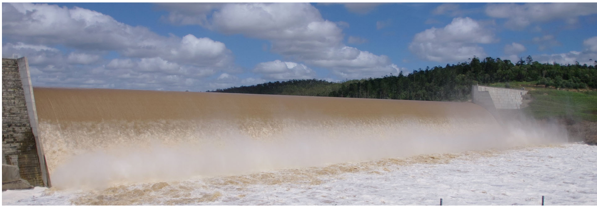
Figure 2. Strong turbulence and intense free-surface aeration in a skimming flow on a stepped spillway. Paradise Dam spillway operation on 5 March 2013 for Q = 2,320 \text{ m}^3/\text{s} , d_c/h = 2.85 , h = 0.62 \text{ m}
