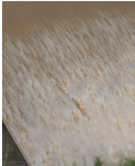
(B) Details of the upper free-surface region during the Paradise Dam spillway operation on 5 March 2013 - Flow conditions: h = 0.62 m, Q \sim 2300 m 3 /s, q \sim 7.4 m 2 /s, d_c/h \sim 2.85 , Re \sim 2.9 \times 10^7
