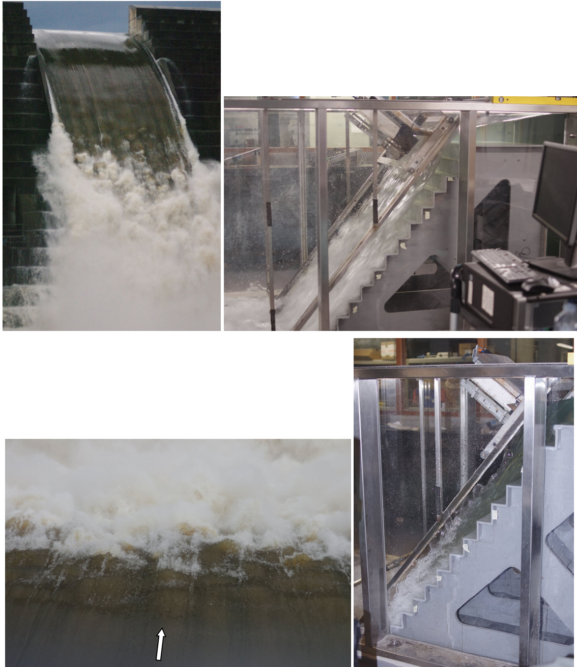
Figure 3. Prototype and laboratory model stepped spillways (1V:0.8H) in operation for d_c/h = 1.6 - Left: Hinze Dam spillway operation on 3 March 2022 (photograph taken under light to heavy rainfall); Right: laboratory model
