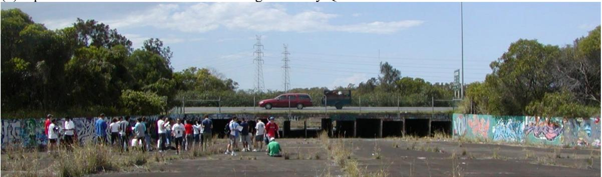
(c) Minimum Energy Loss (MEL) culvert inlet beneath the Gateway Freeway in Wynnum QLD
