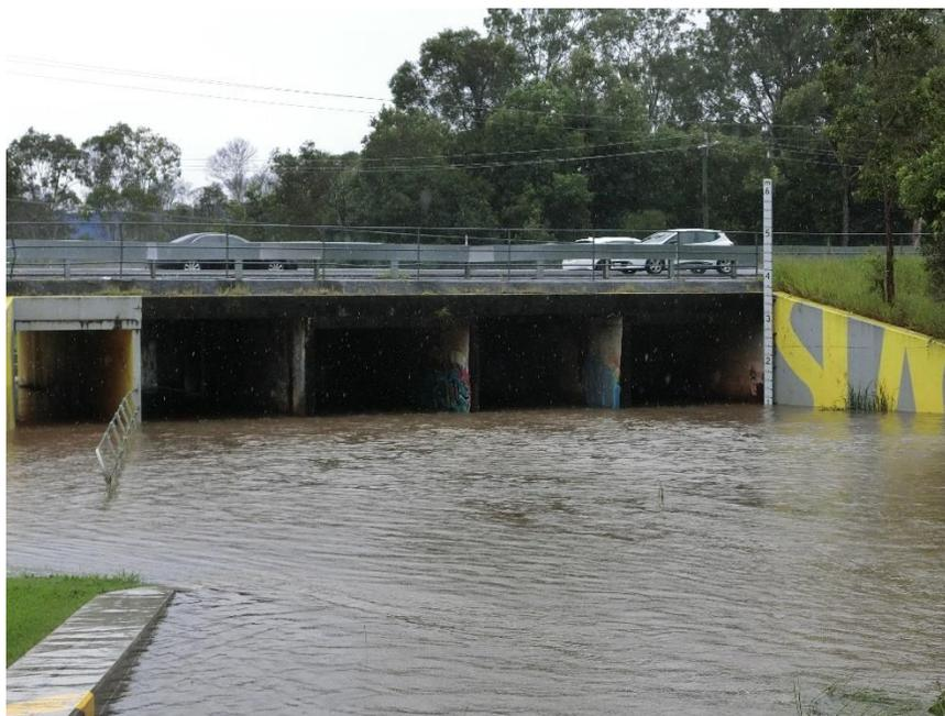
**Figure 2. Retrofitted box culvert outlet with fish-friendly low-flow cell along Slacks Creek in Logan QLD, Australia; in 2018, the estimated cost is \$125,000. Photograph on 22 March 2021 about 14:30 (Photograph Hubert CHANSON)**
