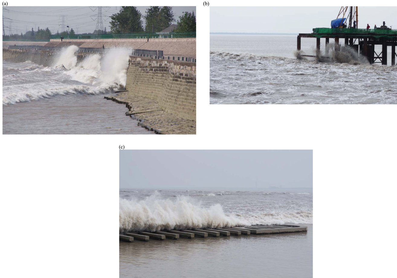
Fig. 1. Photographs of tidal bores impacting man-made structures. (a) Tidal bore of the Qiantang River, China, impacting on an old seawall at Xinchang on 13 October 2014. (b) Tidal bore of the Qiantang River, China, impacting a construction platform at Yanguan on 11 October 2014 — bore propagation from left to right. (c) Tidal bore of the Qiantang River, China, impacting a spur dyke between Yanguan and Laoyanchang on 11 October 2014 — bore propagating from background to foreground, with the bore front impacting the spur dyke on the left. [Colour online.]
