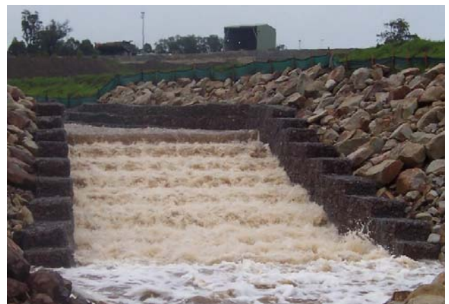
Figure 1. Flow down a gabion stepped weir (Courtesy of Tony Marszalek).
