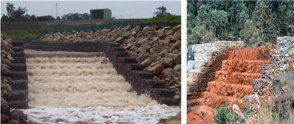
Figure 1. Gabion stepped weirs – Left: courtesy of Tony Marszalek; Right: courtesy of Officine Maccaferri
