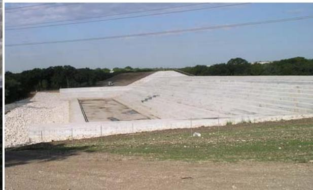
(C) Gold Creek dam stepped spillway on 12 January 2009 (Courtesy of Gordon Griggs) - H = 26 m, h = 1.5 m, 20.6° slope, W = 55 m, concrete stepped spillway completed in 1890
