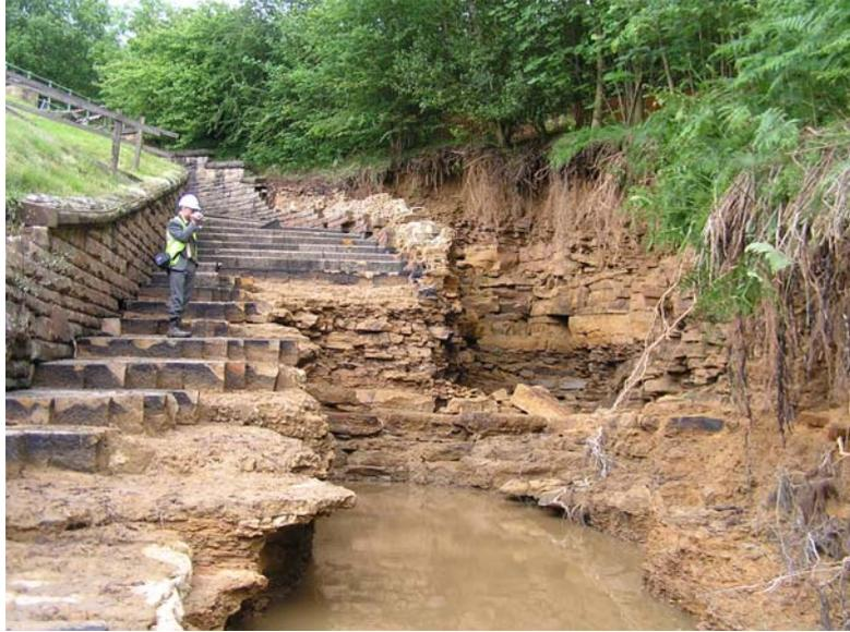
**Fig. 1** - Damaged stepped spillway at Boltby dam (UK) (Courtesy of Peter MASON) - Damage during 19 June 2005 flood, peak flow: 22-30m<sup>3</sup>/s
