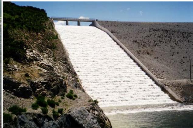
(A) Elkwater Fork dam stepped spillway construction in 2007 (Courtesy of Craig Savelle, USDA-NRCS-NDCSMC) - H = 29 m, h = 0.61 m, W = 46 m, RCC construction completed in 2008
