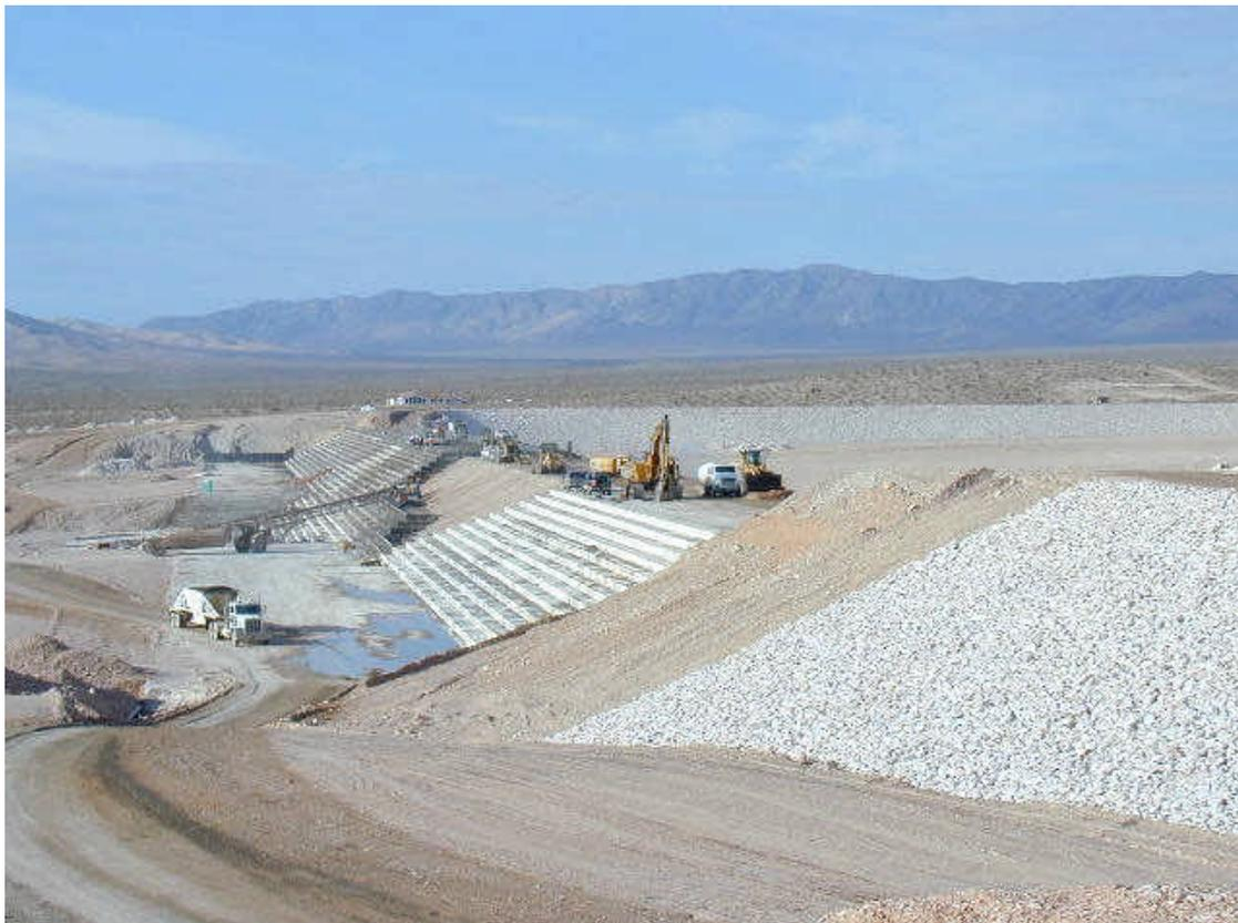
Roller compacted concrete is placed in a succession of overlays of 0.2 to 0.4-m thickness and with a width greater than 2.5 m for proper hauling, spreading and compacting. Exposed RCC is frequently used for secondary spillways with infrequent spills of less than 5 m<sup>2</sup>/s. Alternatively, a conventional concrete protection overlay may be applied after the RCC or at the completion of construction works to
