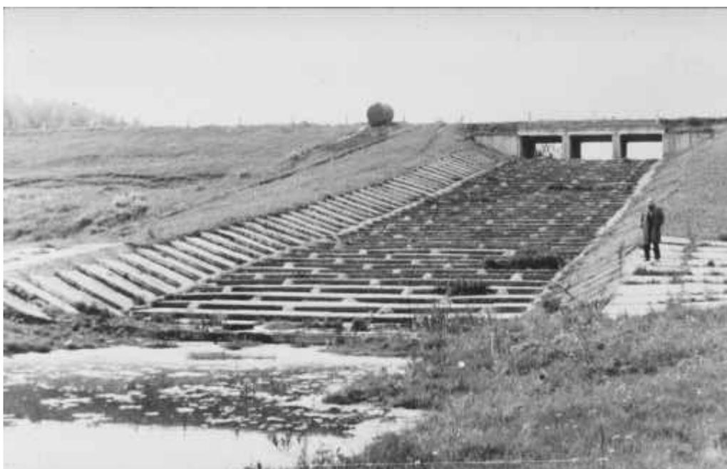
Fig. 7-3 - Earthfill embankment with a rockfill upstream protection and reinforced earth downstream slope construction : Jordan II, Gatton QLD (Australia, 1992) on 22 Feb. 1998 - H = 5.3 m, h = 1.4 m,  $\alpha = 17.7^\circ$  - View from downstream
