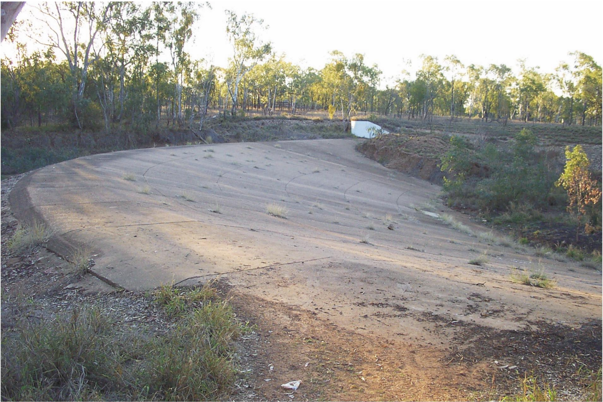
Fig. 2. Minimum energy loss weirs: (a) Sandy Creek weir at Clermont, Queensland, Australia, built in 1963. Dam height = 6.1 m, Q_{des} = 850 \text{ m}^3/\text{s} , B_{crest} = 116 \text{ m} . View from the right bank on 3 September 2002 (courtesy of Keith James). (b) Chinchilla weir, Queensland, Australia, built in 1973. Dam height = 14 m, Q_{des} = 850 \text{ m}^3/\text{s} , B_{crest} = 410 \text{ m} . View from the right bank on 8 November 1997.
