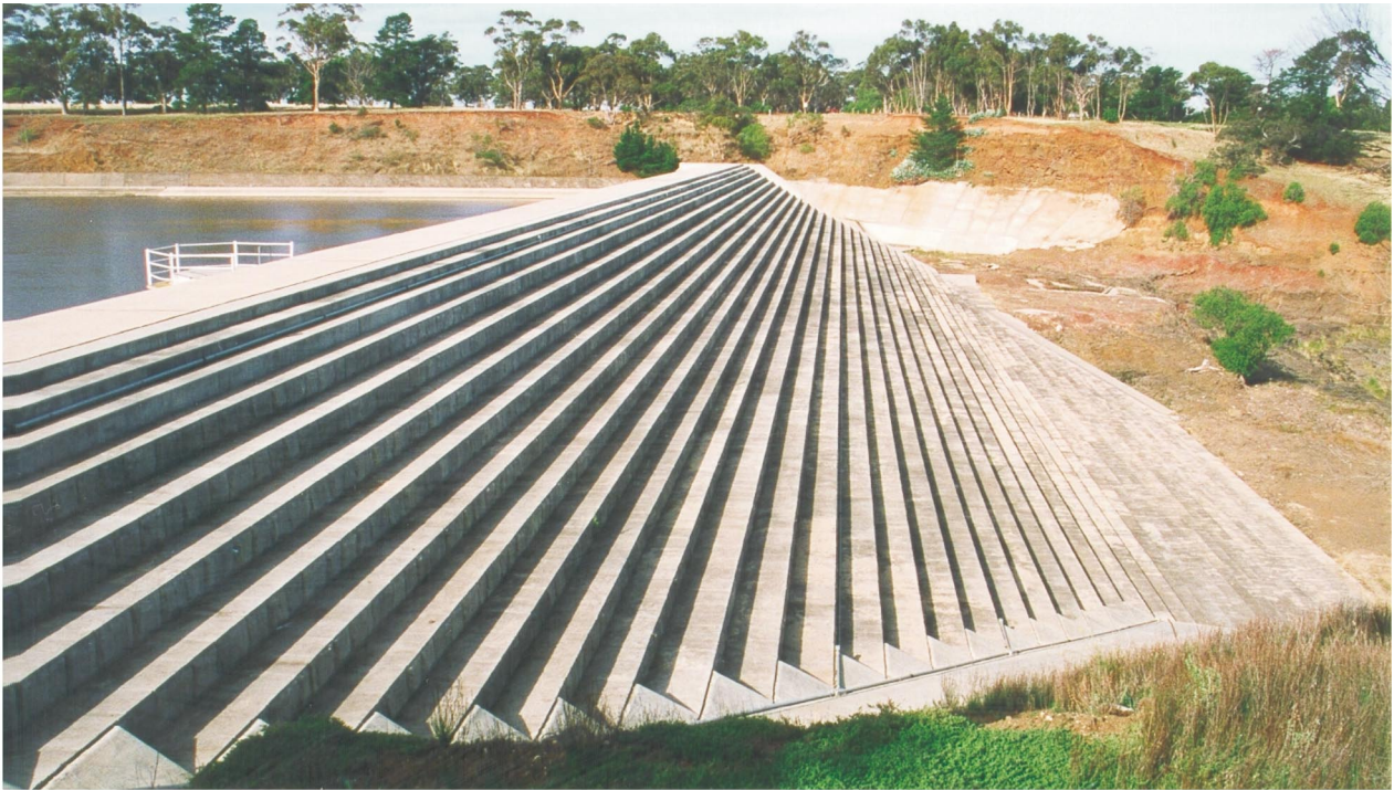
Fig. 1. Embankment dam stepped spillways: (a) Melton dam secondary spillway on 30 January 2000. Completed in 1916, the Melton dam was equipped in 1994 with a secondary spillway ( Q_{des} = 2800 \text{ m}^3/\text{s} , step height h = 0.6 \text{ m} ). (b) Choctaw 8A dam auxiliary spillway (courtesy of Craig Savela and the U.S. Department of Agriculture Natural Resources Conservation Service) ( Q_{des} = 481 \text{ m}^3/\text{s} , h = 0.61 \text{ m} , crest width B_{crest} = 51.8 \text{ m} ).
