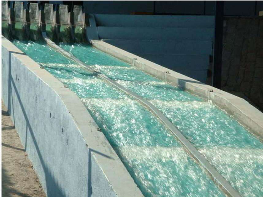
(b) Foz do Areia dam spillway (Brazil) and aeration device in operation (note the air duct intakes) - Note the massive flow aeration from the first set of ducts - Design discharge: 11,000 m<sup>3</sup>/s, Dam height: 160 m
