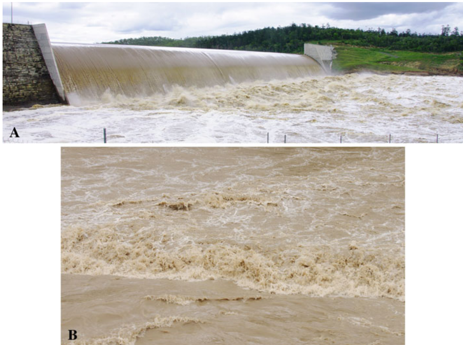
Fig. 1 Photographs of prototype hydraulic jumps. a Hydraulic jump stilling basin in operation downstream of Paradise dam spillway (Australia) on 30 December 2010— Q = 6,300 \text{ m}^3/\text{s} , Re = 1.9 \times 10^7 , b Hydraulic jump during Black Snake Creek flood, Marburg (QLD, Australia) on 11 Jan. 2011—flow from foreground left to background left , looking downstream
