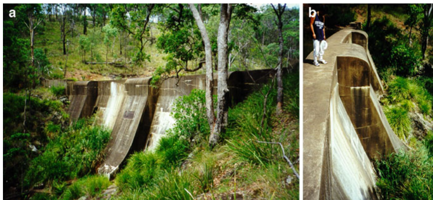
Arch Dams, Development from Cut-Stone Arches to Modern Design, Figure 4 75-Miles dam (Warwick QLD, Australia). (a) View from downstream of the dam with the three concrete buttresses (Photograph taken on 23 January 1998). (b) Details of the dam crest and buttresses (Photograph taken on January 23, 1998).
