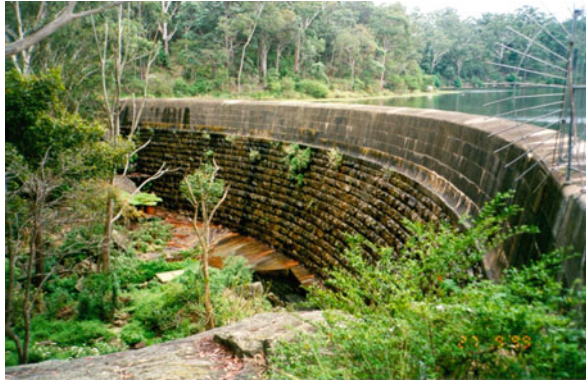
Arch Dams, Development from Cut-Stone Arches to Modern Design, Figure 3 Parramatta dam, Sydney, Australia on September 27, 1999.
