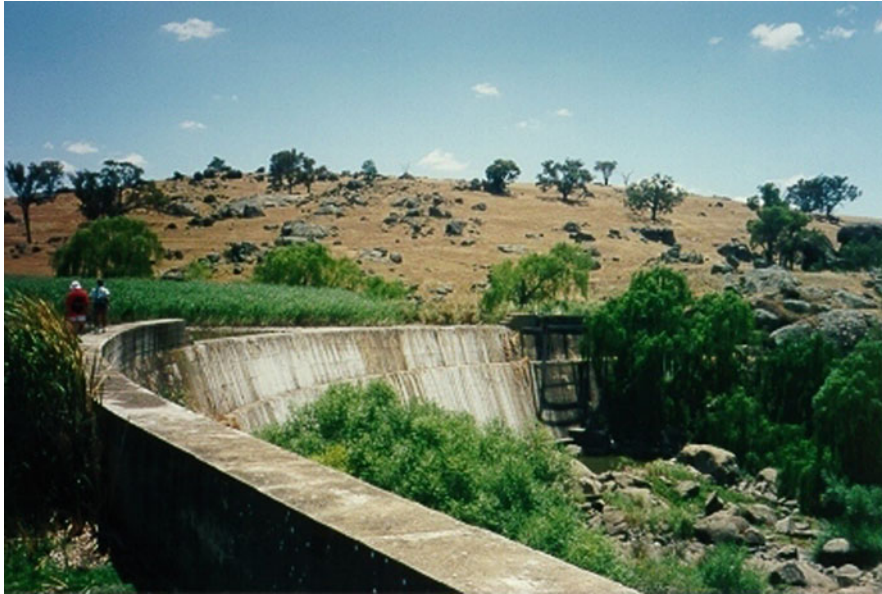
Reservoir Sedimentation in Australia under Extreme Conditions, Figure 3 Fully silted reservoir of Cunningham Creek railway dam (Harden NSW) completed in 1912 – view from the right bank in December 1997.
