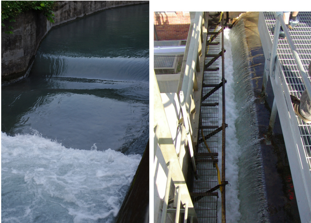
(A, Left) Hydraulic jump in an irrigation channel on 10 November 2010 in Hualien County (Taiwan) - Flow from top right to bottom left (Shutter speed: 1/100 s)
