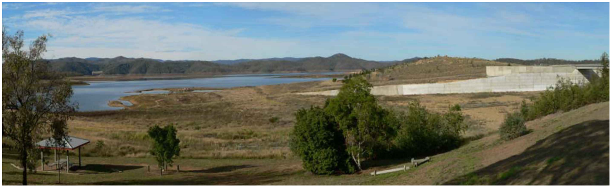
(A) Dry reservoir on 13 June 2007 viewed from the dam right abutment with the secondary spillway intake on the far right - The reservoir capacity was below 16%.
