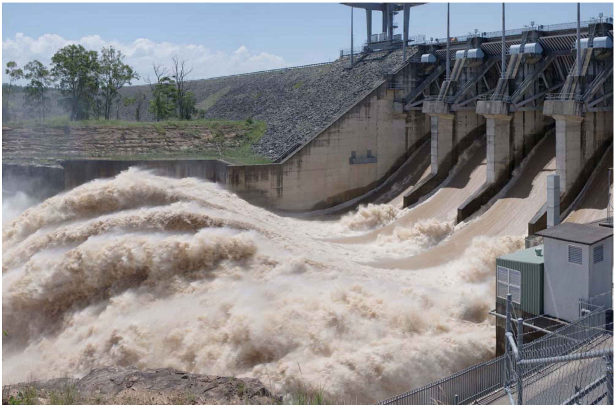
(B) Spillway operation on 17 January 2011 - The reservoir capacity was about 122%.
