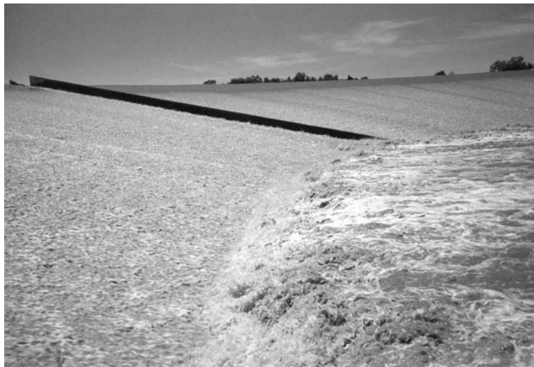
Figure 1. Air entrainment at Chinchilla weir (Australia) – Note self-aeration down chute and in hydraulic jump (foreground) – The beige colour of water is caused by three-phase mixing (air, water & sediment).
