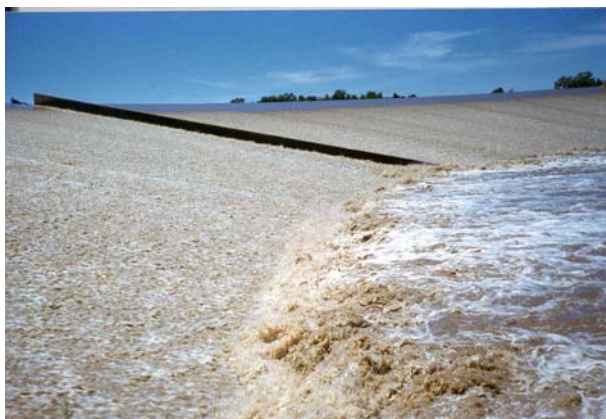
(C) Chinchilla weir (Qld, Australia 1973) - Small overflow view from the right bank on 8 Nov. 1997
