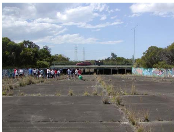
(C) Inlet of MEL culvert in Wynnum North, Brisbane in Sept. 2002 - Note passing cars on Gateway motorway and undergraduate students in inlet
