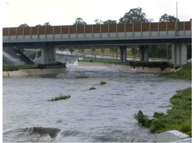
(D) Minimum Energy Loss waterway in Brisbane - Outlet operation on 31 Dec. 2001 for about 80 \text{ m}^3/\text{s}
