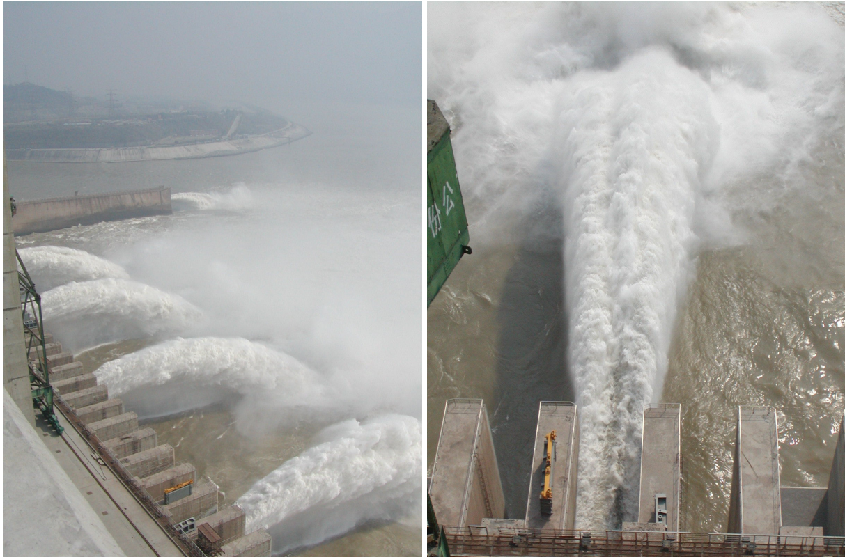
Fig. 1 Photographs of air-water flow at bottom outlet - Three Gorges Project on 20 October 2004, V_0 = 35 m/s, Q = 1700 m 3 /s per outlet, W_0 = 9 m (per outlet)
