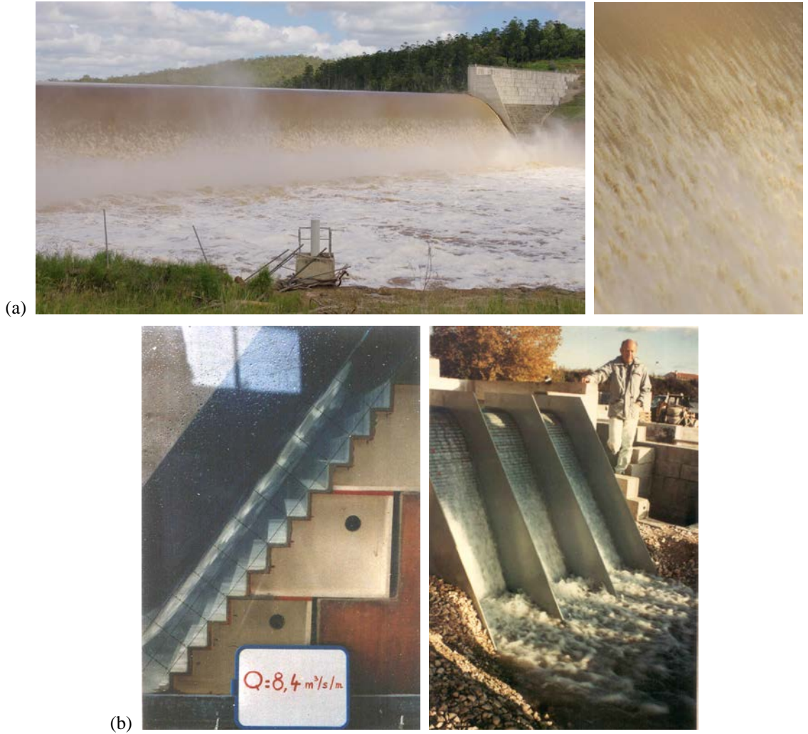
Figure 1 Comparison of air-water flows between prototype and laboratory model operations of stepped spillways; (a) Paradise Dam stepped spillway (Australia) in operation on 5 March 2013 (Photographs H. Chanson): Q \approx 2,500 \text{ m}^3/\text{s} , h_c/h = 2.9 , R = 7 \times 10^6 , h = 0.62 \text{ m} , \theta = 57^\circ - View from downstream (left) and details of air-water flow structures next to the inception point of free-surface aeration (right); (b) Laboratory experiments (Courtesy of Mr P. Royet, IFSTTAR) – Left: Q = 0.40 \text{ m}^3/\text{s} , h_c/h = 3.2 , R = 2.6 \times 10^5 , h = 0.060 \text{ m} , \theta = 53^\circ ; Right: R < 4 \times 10^4 , h = 0.024 \text{ m} , \theta = 63.4^\circ, 59^\circ \& 53^\circ (from left to right)
