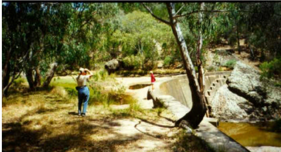
Fig. 4 - Cunningham Creek dam, Harden NSW, 1912 (Photograph on 28 December 1997)
