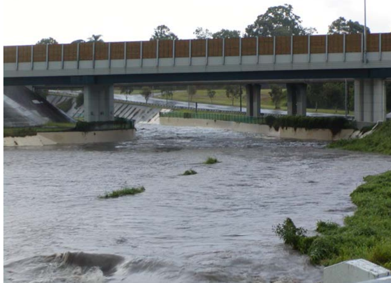
(B) MEL waterway in operation on 31 Dec. 2001 for about 80 m 3 /s looking upstream
