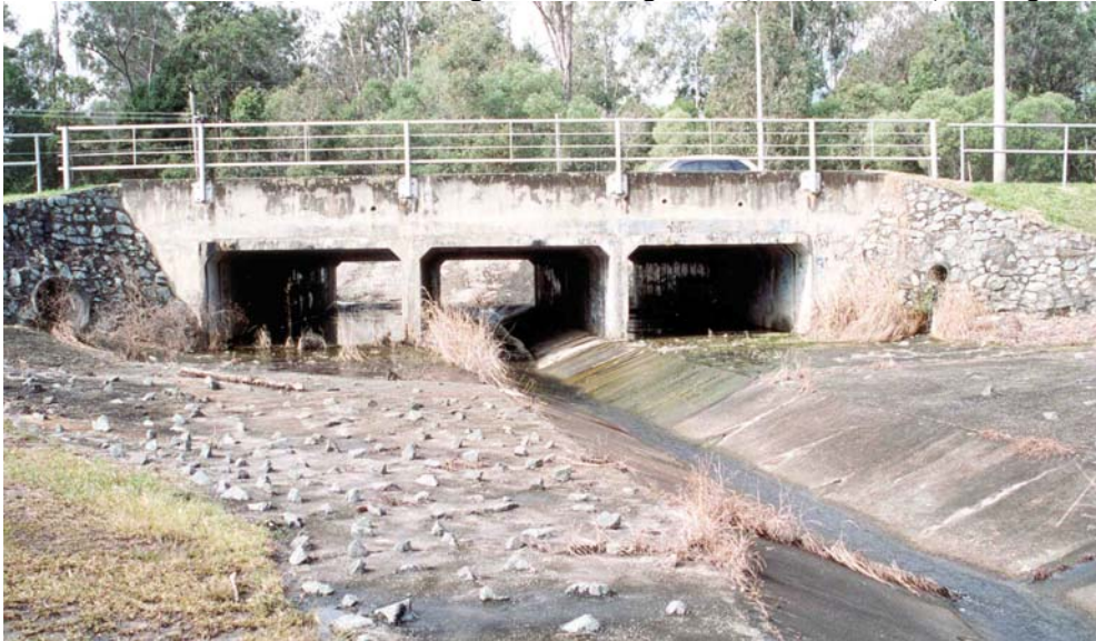
Fig. 2-1 : Standard culvert outlet below Algerster Rd, Algerster QLD (Australia) in Aug. 1999
