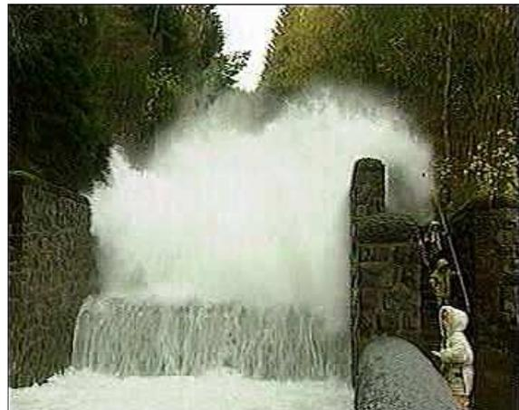
(A) Free-surface instability propagating down the Sorpe dam spillway (Germany) on 2 November 1998 (Courtesy of Ruhrverband) -  $\theta \approx 18^\circ$ ,  $h = 0.5$  to  $2$  m,  $Q = 6.9$  m<sup>3</sup>/s,  $Re = 1.0 \times 10^6$  - Note the children on the foreground right
