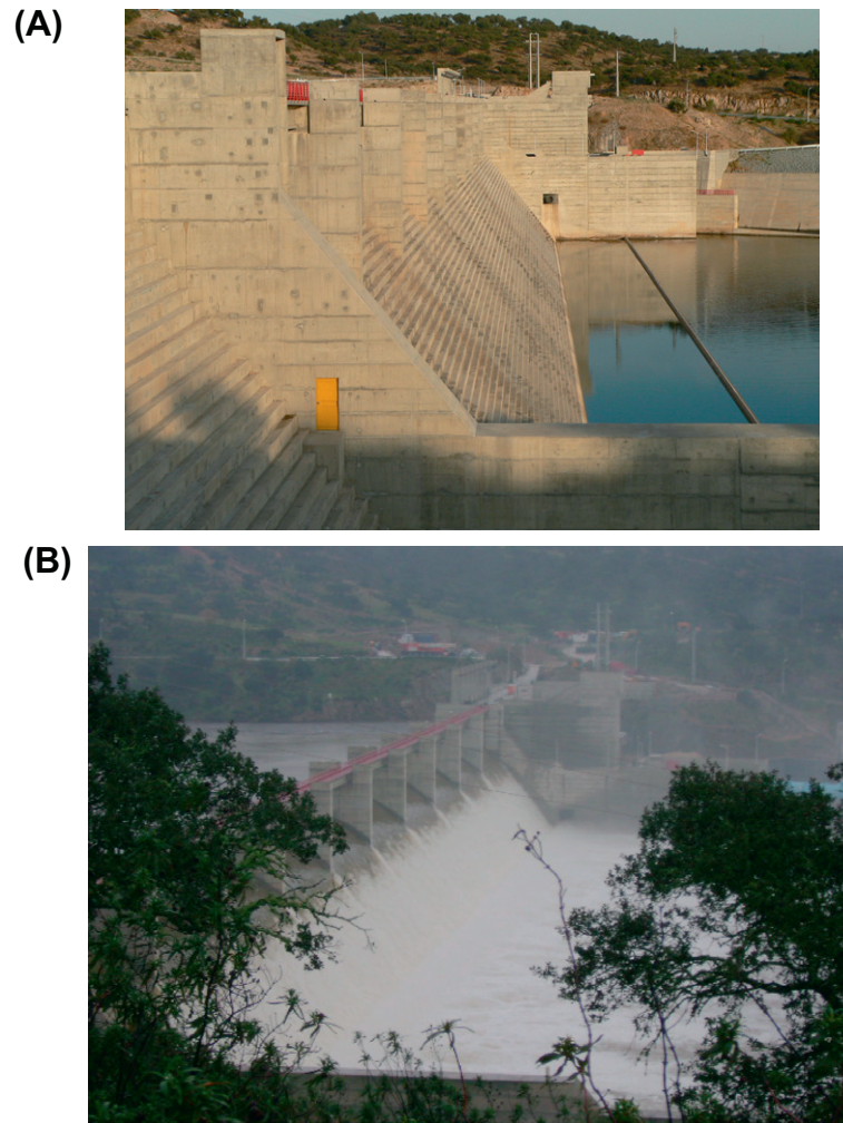
Fig. 1. Pedrogao dam stepped spillway (Portugal) – Roller compacted concrete gravity dam ( H = 43 m, L = 473 m), uncontrolled overflow spillway ( W = 300 m, h = 0.6 m, \theta = 53.1^\circ ). (A) Stepped spillway on 4 September 2006. (B) Skimming flow on 16 January 2010 with a discharge 1000 \text{ m}^3/\text{s} , Re = 1.3 \times 10^7 (Courtesy of Professor Jorge MATOS).
