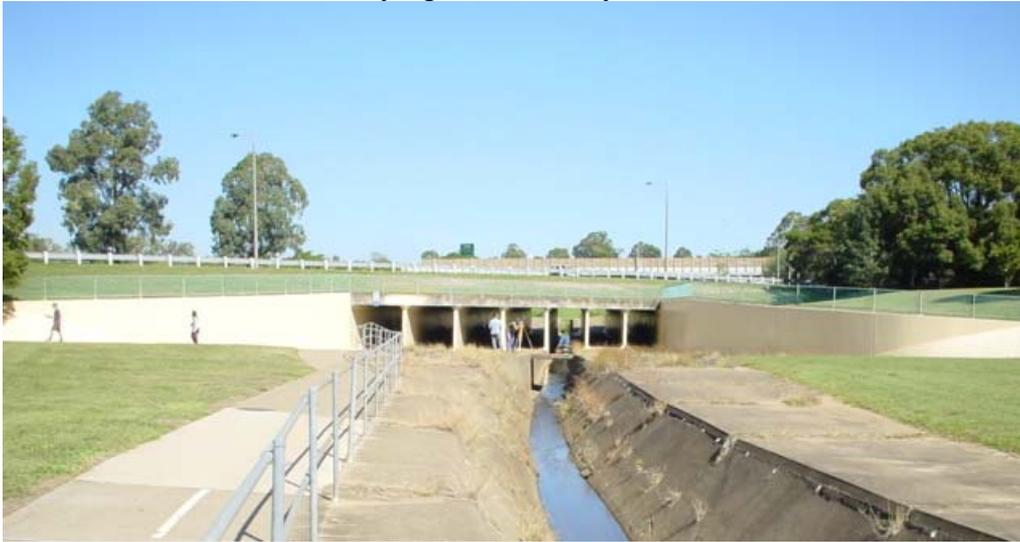
(B) Culvert outlet in operation on 31 Dec. 2001 for about  $80 \text{ m}^3/\text{s}$  (flow from left to right)
