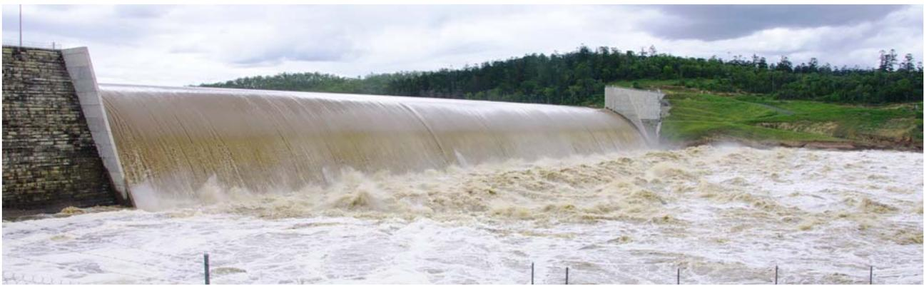
Fig. 1 - Hydraulic jump stilling basin in operation downstream of Paradise dam spillway (Australia) on 30 December 2010 -  $Q = 6,300$  m<sup>3</sup>/s,  $Re = 1.9 \times 10^7$
