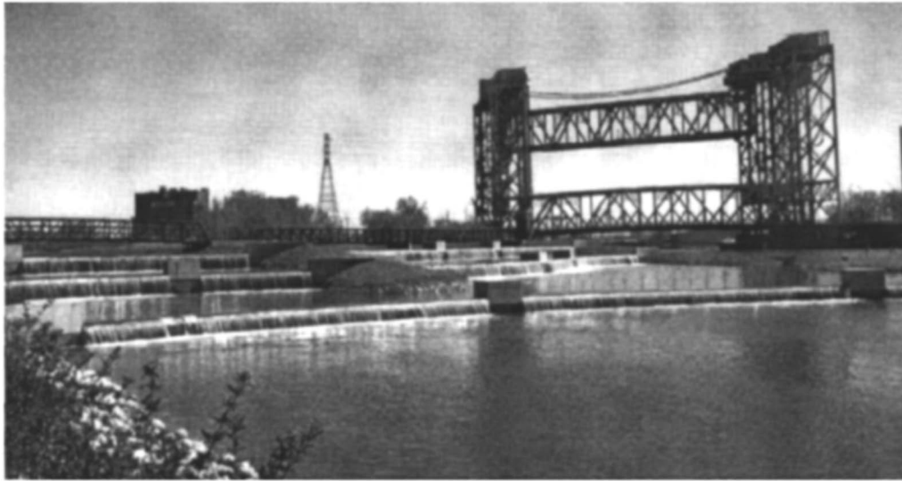
Fig. 1. Sidestream elevation pool aeration cascade (Chicago, Ill. 1988) (courtesy of The Metropolitan Water Reclamation District of Greater Chicago, with permission)
