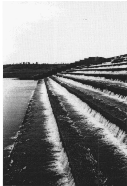
Fig. 2. Rockfill stepped weirs: (a) Rockfill stepped weir made of Reno mattresses in Robina, Gold Coast, Australia; and (b) Gabion stepped weir at Guaribraba, Capo Grande, Brazil (Courtesy of Officine Maccaferri)—note the seepage flow, the absence of overflow, and the increasing seepage with downstream distance from the crest
